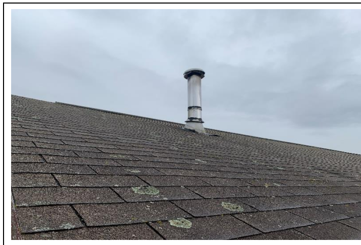
6. Seam sealant on chimney – Assumed ACM
